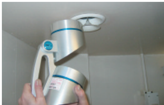
Check of air duct before cleaning
